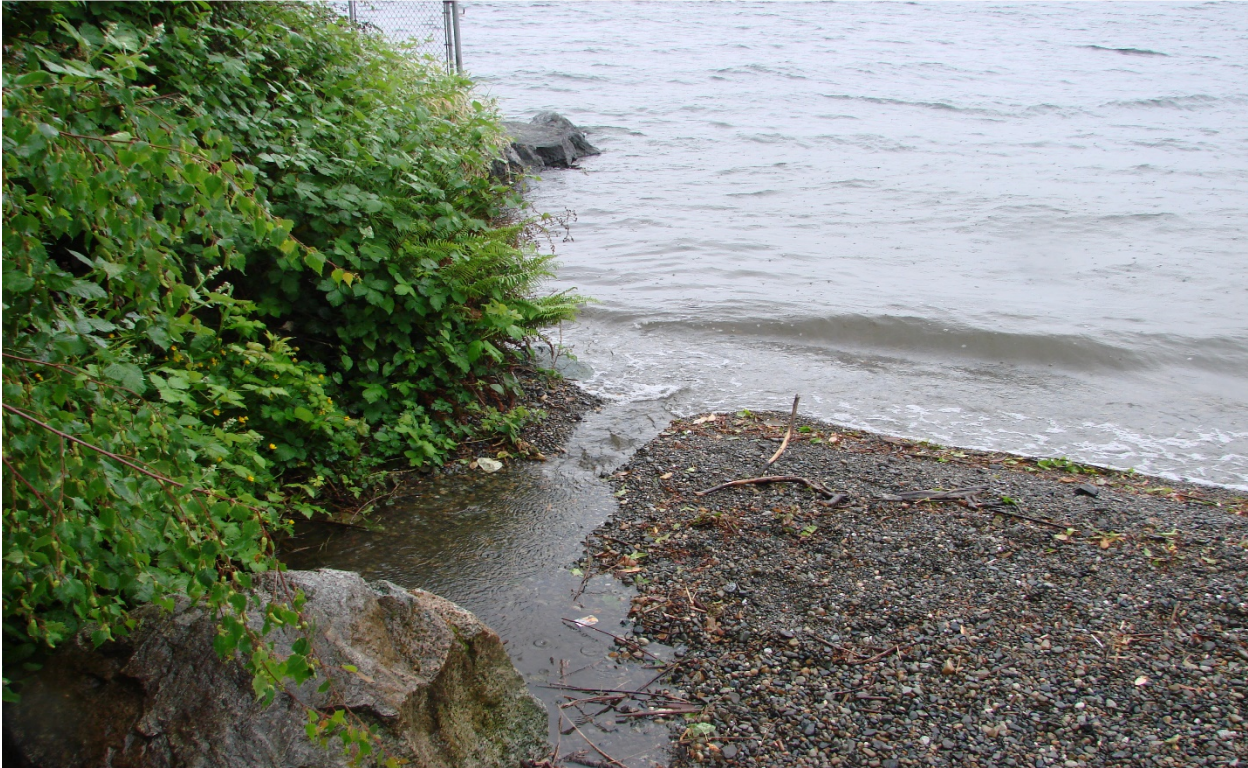
Photo #13 – Outfall into Lake Washington at beach head
